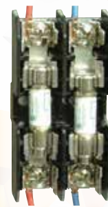
Defrost Heater Fusing
